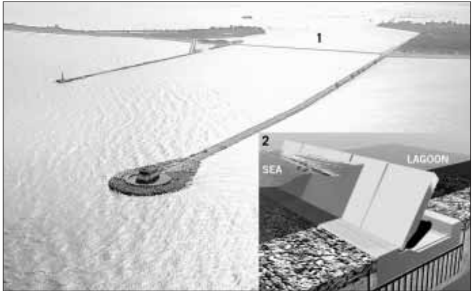
Perspective diagram of the Malamocco opening (1) and a second diagram (2) showing some of the gate segments in a raised position.
