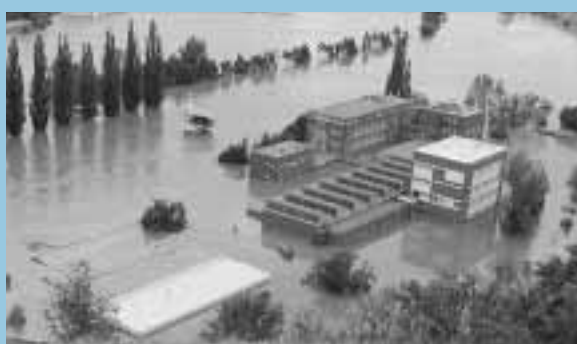
Library of the Water Research Institute in Prague, Czech Republic completely flooded (August 2002).
