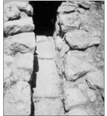
Fig 1. Exit of the main sewage collector of the palace of Cnossos (Crete). About 80 cm high and 40 cm wide (photo by the author).
