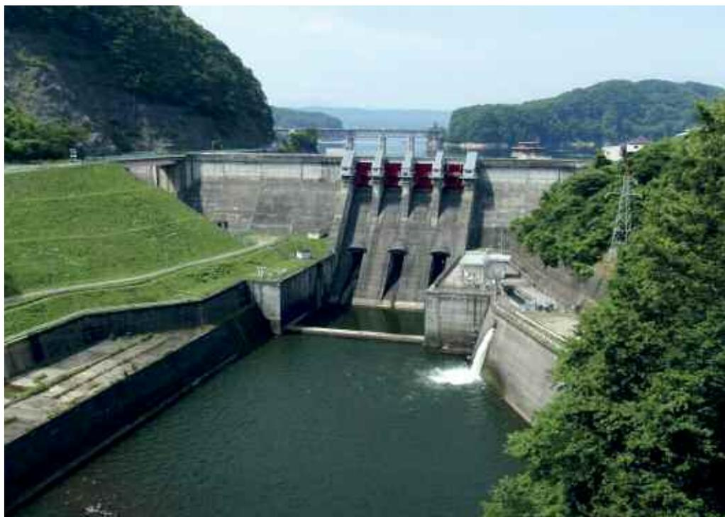
Figure 1. Kamafusa Reservoir, a multi-purpose reservoir operated for flood control, water supply and power generation in the Natori River basin in Japan. The reservoir provided enhanced capability for flood protection by introducing prior release operation considering real-time hydrological predictions while river levees in the downstream were damaged by the great earthquake and tsunami in 2011
